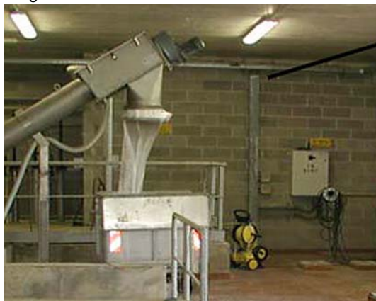
VERSA Drum Screen fitted with screenings bagging system discharging to a container
